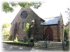
St Richard's Parish, Skelmersdale
